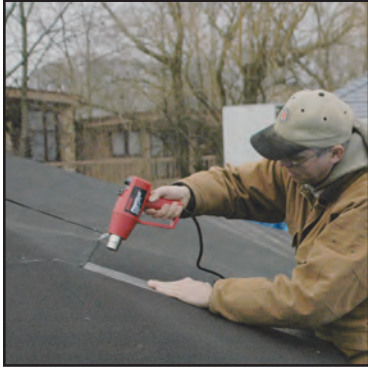
Weld Roofing Membrane
